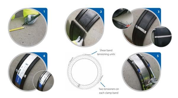
**Preparation:** Remove deposits and dirt from the pipe. Select a point as close as possible to the apex of the pipe where the pipe crack or damaged area has the smallest gap or no gap at all. The gap must not exceed 20 mm.
