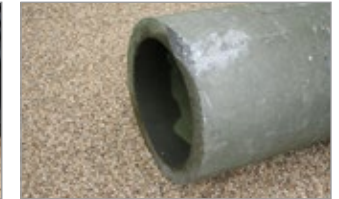
Pipes with a damaged surface
